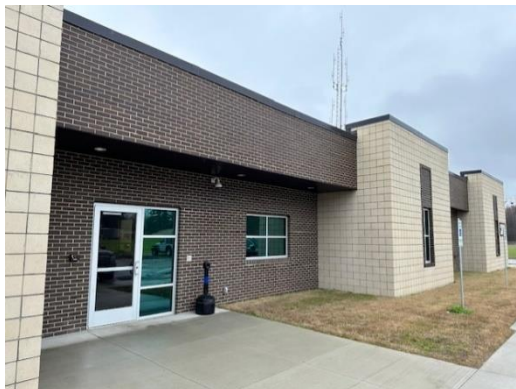
St. Francis County 9-1-1 October 1, 2022
